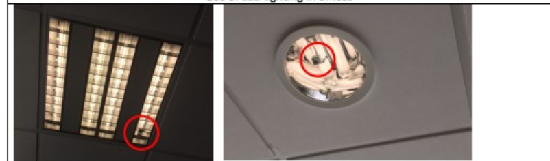
Use of energy saving lamps with light detection (less electricity is used by lamps when daylight is sufficient).
