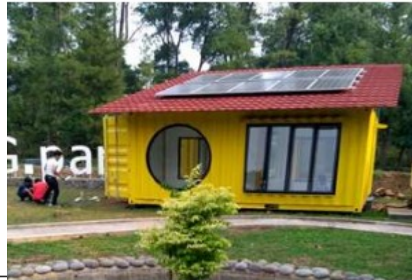
Solar Power Plant of Engineering Park Faculty of Engineering
